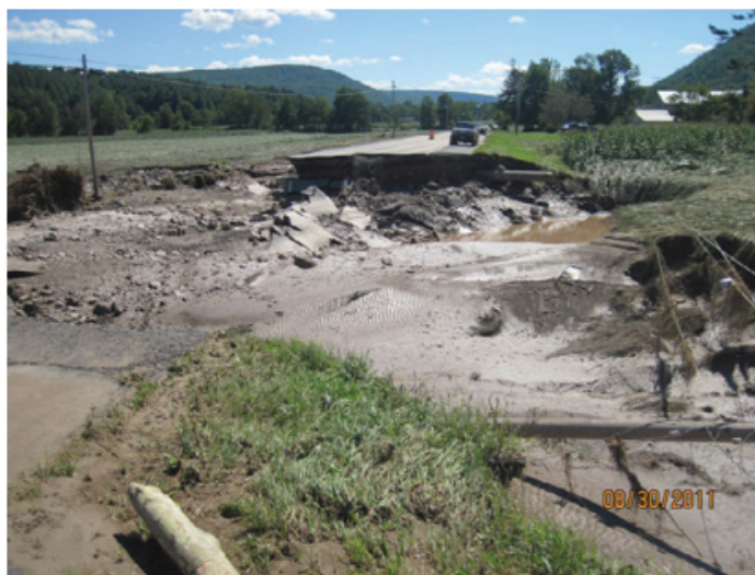
Flood of August 2011, State Route 30 road washout caused by Schoharie Creek at Breakabeen, New York. Photo by Joseph Griffin, courtesy of New York State Department of Transportation (USGS 2014).
